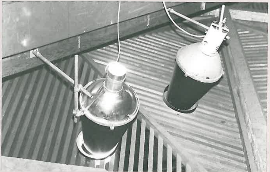
A detail showing the original and modified lighting fitting taken from the walkway above the suspended ceiling, and a section of one of the luminaires.
